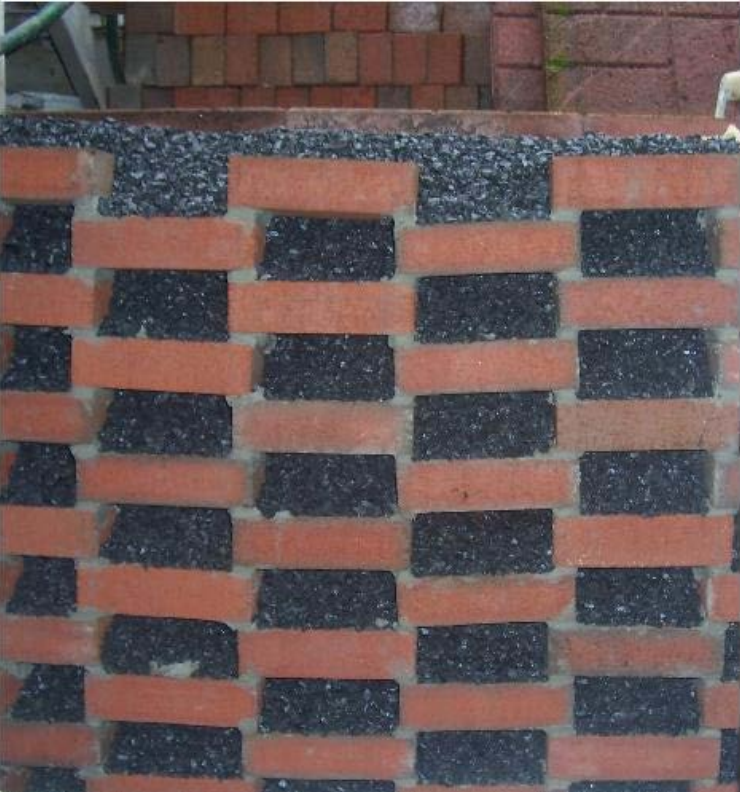
Particular Wall™ made of Bricks (Window Well Retaining Wall Application -- 801 Fairway Road State College, PA)
